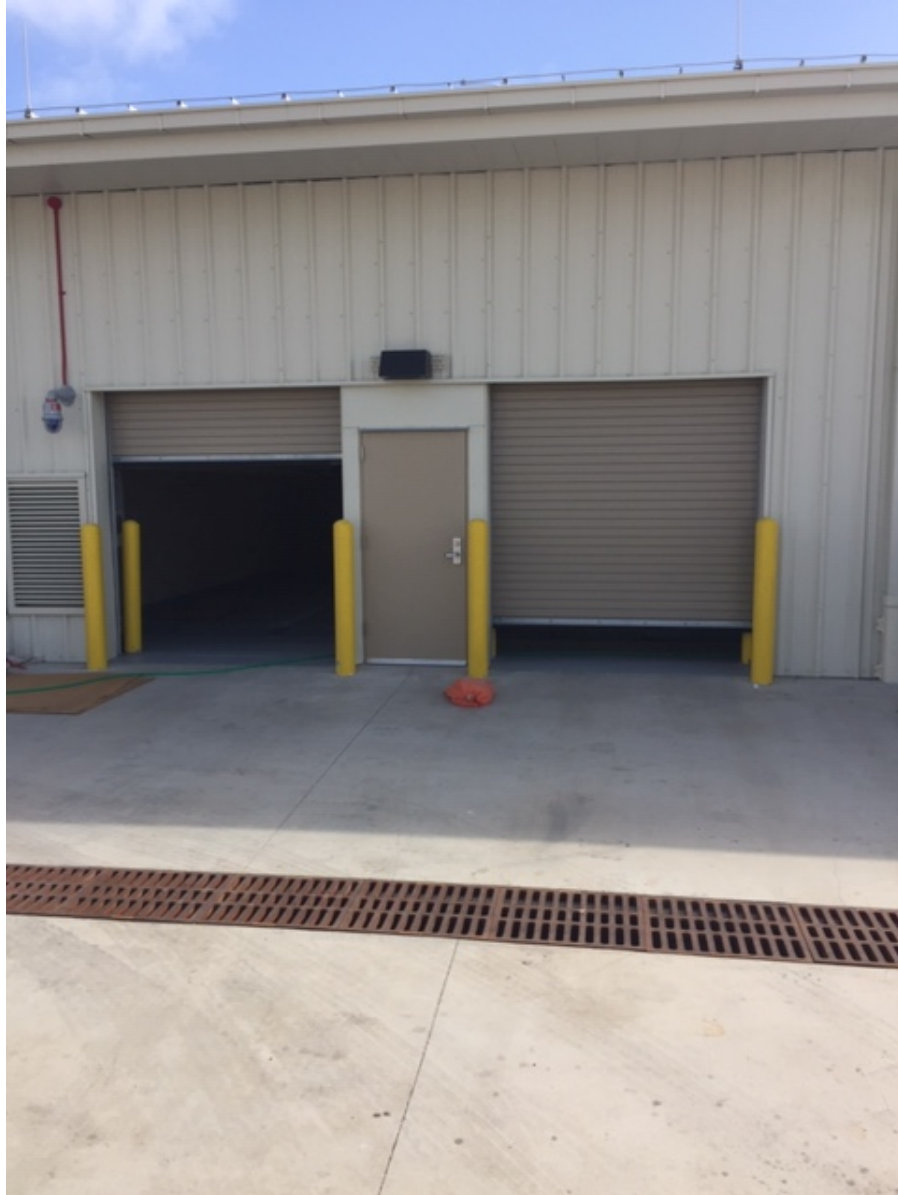
Exterior area around hazardous waste storage bays
