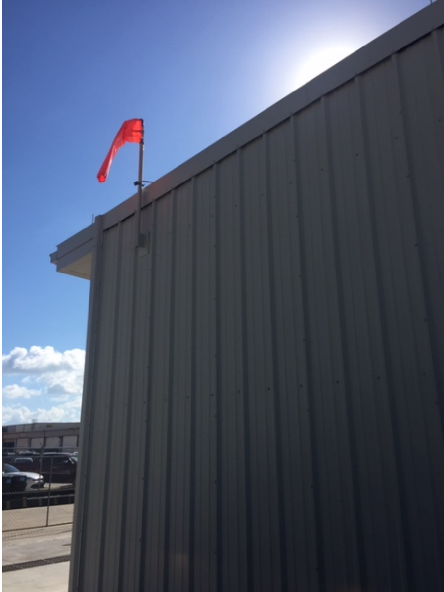
Wind sock on building exterior.
