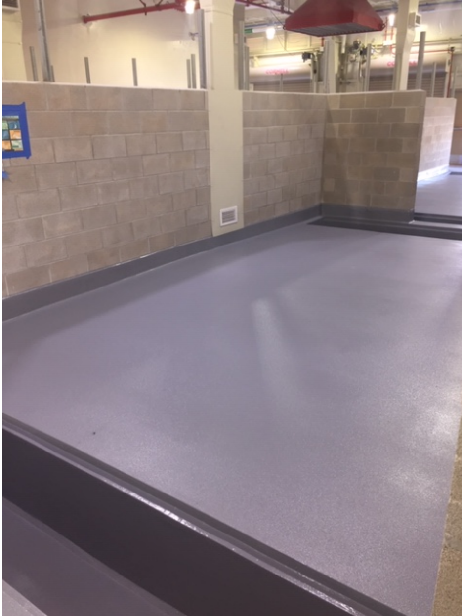
Hazardous waste storage bay with final floor finish
